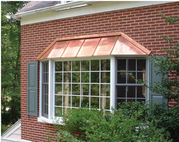
Chapman Windows and Doors installed this SEMCO bay window in place of a flat combination double-hung unit. The copper roof was also built on-site.
