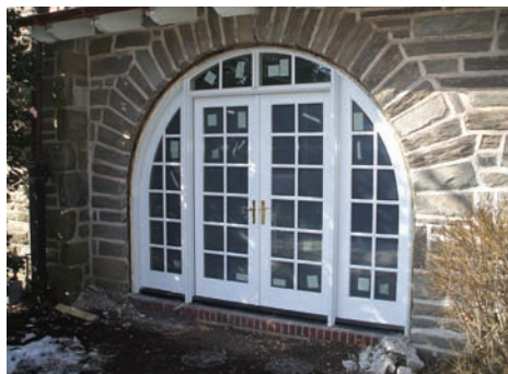
Chapman Windows and Doors installed this SEMCO window and door combination unit to replace an old wood unit in the stone opening.
